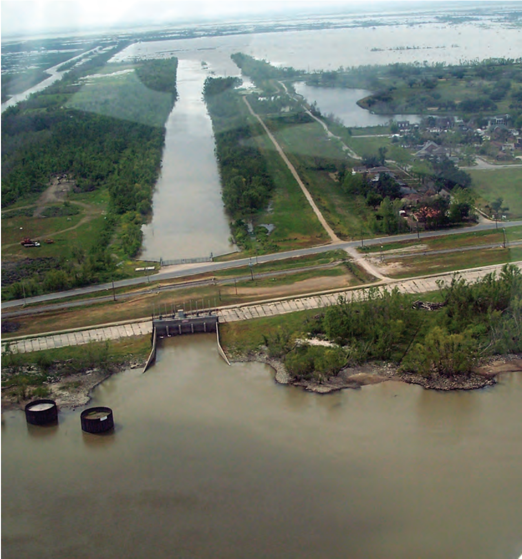
FIGURE 13.10 The Caernarvon Diversion structure on the Mississippi River allows floodwaters to pass through an artificial levee and enter the wetlands of Breton Sound in the distance. (Courtesy J. Day.)
